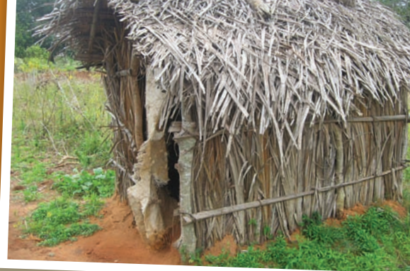
Recently built latrine from local material.
