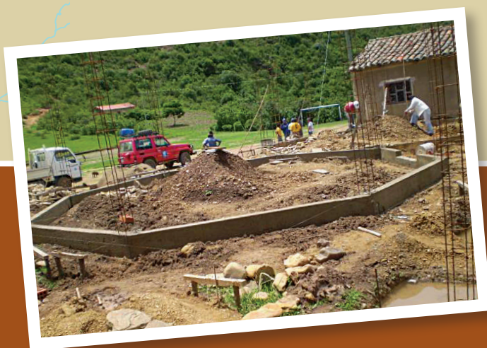
The foundation of a school being built.
